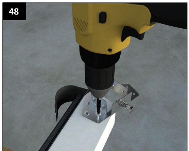
Fix the adjustable glazing ridge bracket to the aluminium glazing bar side of the "A" frame on the ground using 4 x NRTS100 screws.
