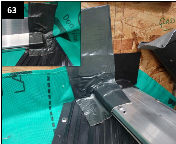
63 Image shows examples where 1 Butyl patch is applied – Glazing on duo-pitch segment (main image) and glazing on lean-to segment (inset image)
