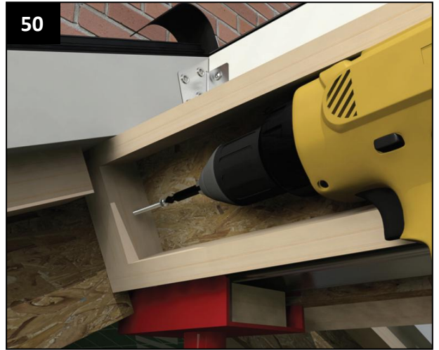
50 The glazing bar should rest on top of the purlin as shown. Pull the purlin towards you to fully engage with ridge hook feature. Screw sideways into the panel edging as shown (BPS025 screw) ...
