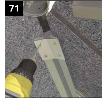
71 Fix the internal upper hip brace plate using 4 x CHAA 006 screws provided.
