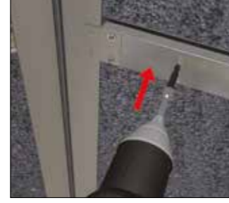
Fixing internal clips
