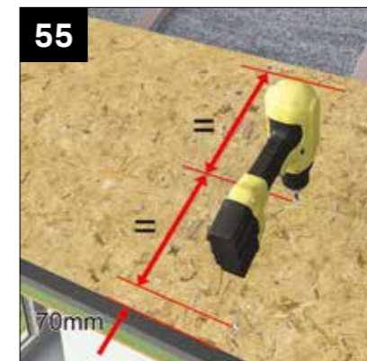
With OSB in position fix board 70mm up from tile starter support and 70mm down from upper edge followed by 1 x central fixing. NOTE: Fixing position at step 56.
