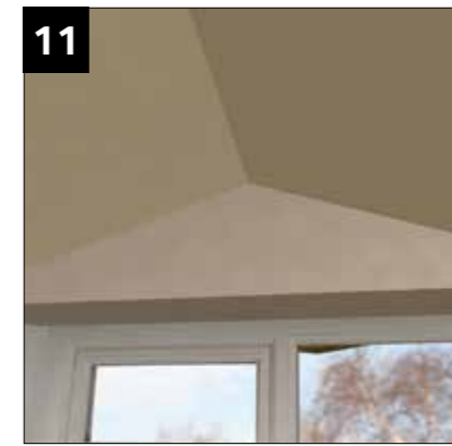
11 Plasterboard face of gable
