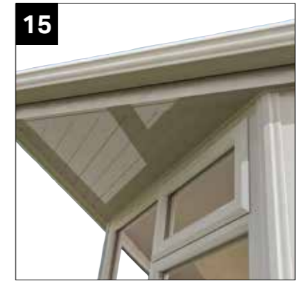
15 Cut and fit ship lap to suit.
