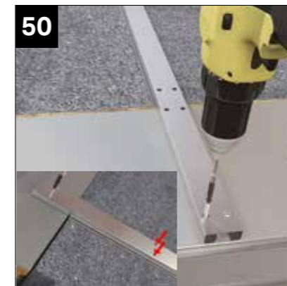
Finally secure the external clips using WPCS020 4.8mm x 38mm self drilling screws provided. (2 into ridge section, 4 into panels and 4 into box beam on full length clips) or through pre-drilled holes on short clips or half clips.
