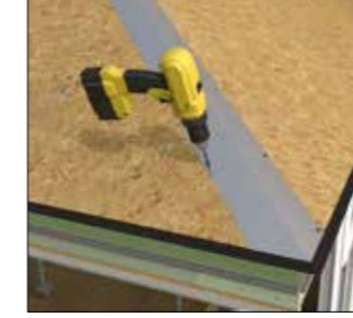
Fixing steel hip plates
