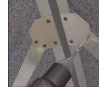
Fixing internal jack rafter connection plate
