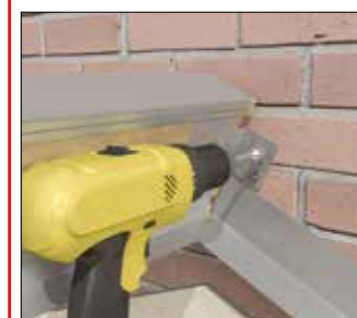
Fixing ridge bracket
