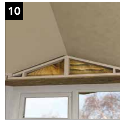
10 Insulate void with mineral wool.
