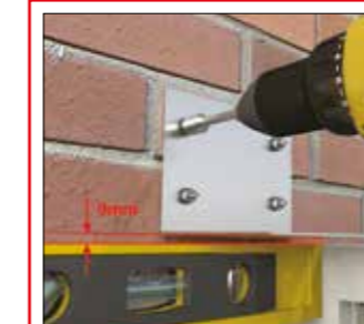
Fixing hanger bracket to wall
