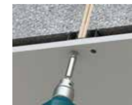
Dry wall bit assembly
