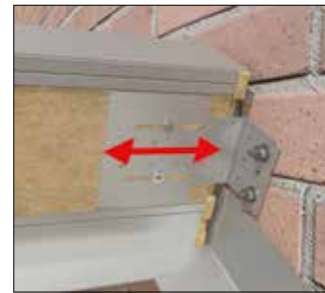
Fixing ridge bracket
