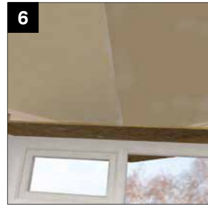
6 Plasterboard the roof.
