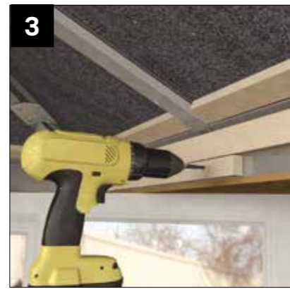
3 Attach additional battens.
