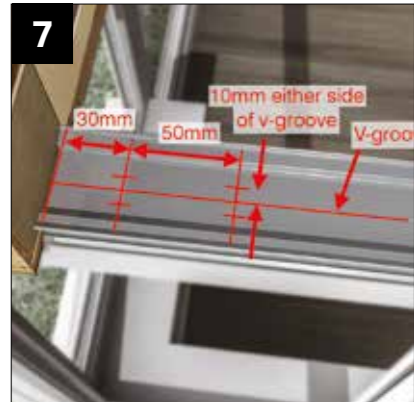
The 4 fixing positions.
