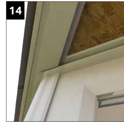
14 External ship lap cladding edge channel detail.
