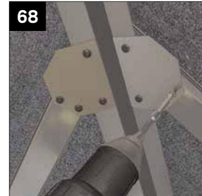
68 Where jack rafter abuts hip bar fix the jack rafter connection plates using 4 x CHAA 006 screws provided. NOTE: fit one screw through half clip that meets hip bar.
