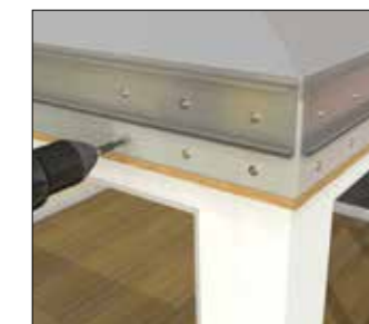
Securing corner cleats
