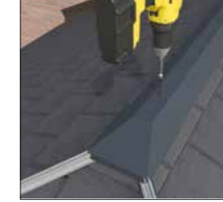
Fixing ridge top cap
