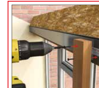
Fixing support props to beam
