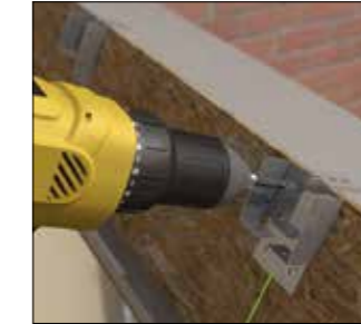
Fixing glazing bar shoes at box beam
