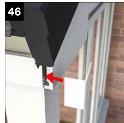
46 Fit 90° external corner cover trims
