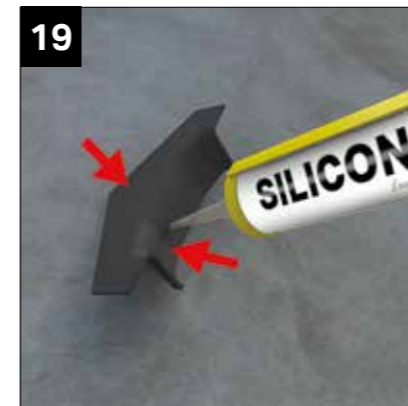
19 Apply clear low modulus silicone to the faces shown and refit.
