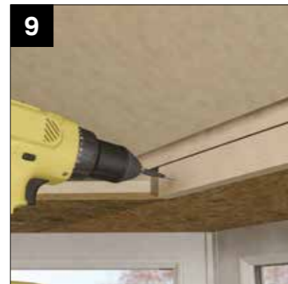
9 Attach additional mating timber battens.
