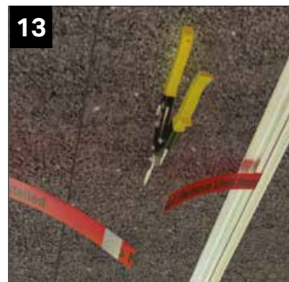
With the expandable panel in position, snip all the retaining straps.
