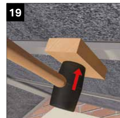
Now offer into position the pre-drilled internal panel clips. Again, use timber packer to prevent indentations to the internal clip. NOTE: short lengths, tap into position. Longer lengths, follow sequence steps 22-24.
