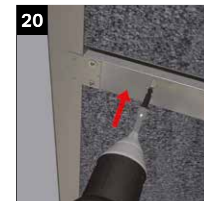
Firstly secure into the panel (at the ridge end) using dry wall fixing screws WPDS020 NOTE: See method of alternate tightening as shown 22 to 24.
