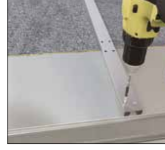
Fixing external clips
