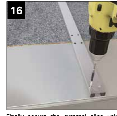
Finally secure the external clips using WPCS020 4.8mm x 38mm self drilling screws provided. NOTE: do not stand on the panels to secure the external clips. Tip: on greater projections secure the clip to the beam (as step 16). Then fit the first row of OSB boarding, this will allow easier access to secure the panel clips further up the roof.
