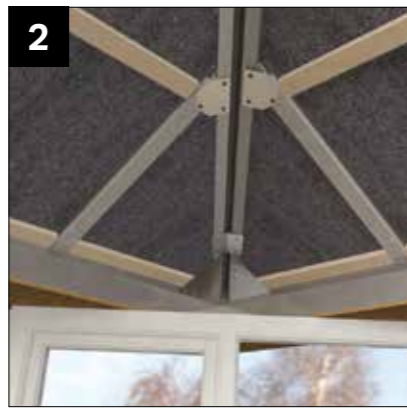
2 Batten out to suit plasterboard fixing.
