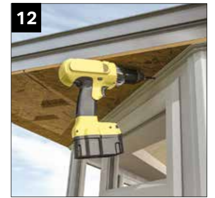
12 Fit external soffit channeling.
