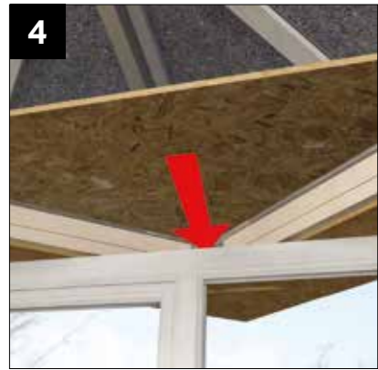
4 Slide into position additional external OSB board.
