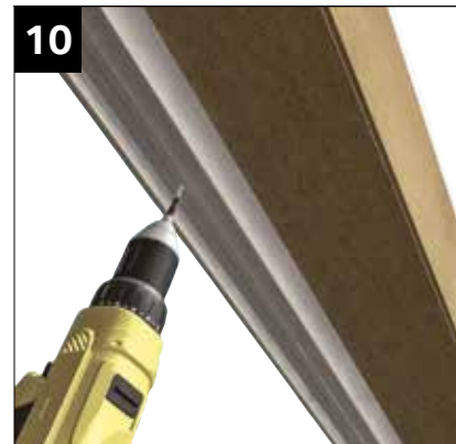
After checking the correct overhang secure the gable panels by screwing up through the head of the frames. Fixings need to be within 200mm of each corner (dependant on access) and at 450mm centres using for example, 4.8mm x 80mm screws; not supplied.
