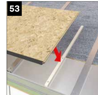
Where required support OSB board at butt joints using timber battens supplied. Battens are 65 x 19 x 700mm long (NRPB010). Only required over box beam using the screws provide WPCS 020 (2 x per batten).
