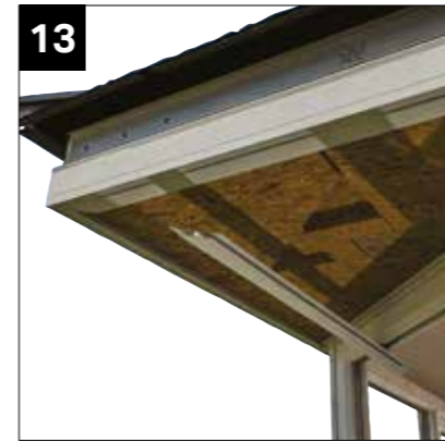
13 Fit external ship lap cladding edge channel.
