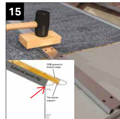
When aligned (ensure external panel clip butts upto aluminium gutter channel, see red arrow) use a robust mallet to knock down the external panel locking clips (use a short length of timber to protect the clip from indentations).
