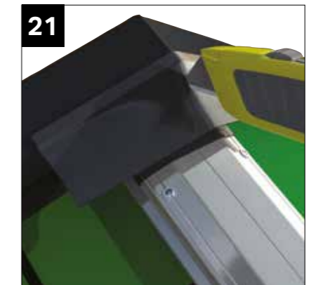
21 Fit second 200mm Butyl tape sealing the dry verge to the gable flashing. Cut the tape to allow it to be folded as shown in the following two images
