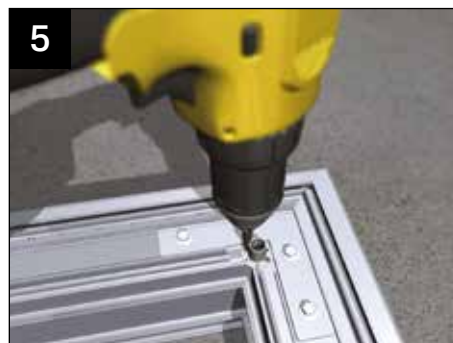
5 If supplied, fasten to each corner the tie bar drop rod fixing bracket to the underside of the lantern eaves beam.
