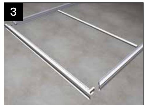
3 Layout the pieces of the lantern eaves beam.
