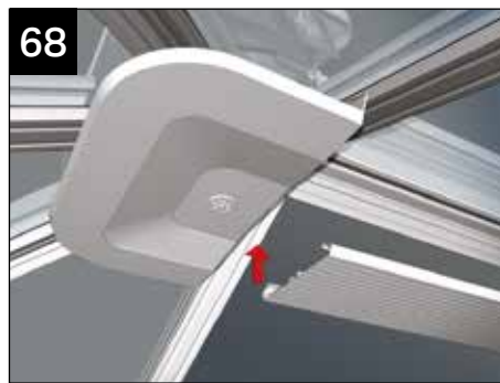
Clip the internal ridge cladding onto the underside of the ridge.
