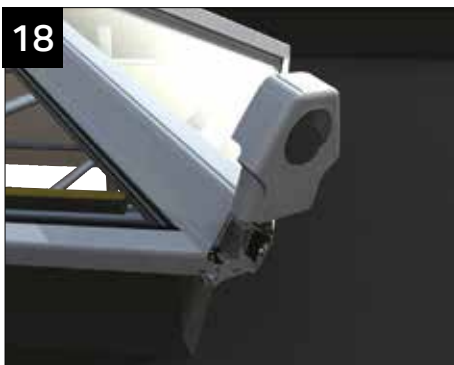
18 Fit end caps to bars and push in circular cover disk to finish.
