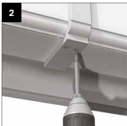
Whilst ensuring that the jointer remains located in position, screw fix using self drilling screws CRN007.
