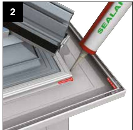
2 Silicone seal front and back edge of lower Cornice sections (be generous). Similarly butter 'DAM' sealer - position within 50mm of any stop end or outlet.
