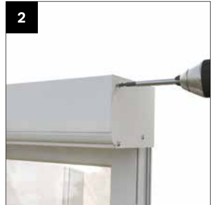
GUTTER STOP END DETAIL - Used with lean-to roofs, gable roofs or when then gutter returns along the host wall. Secure the end plate into position using the fixings provided (CRN008).
