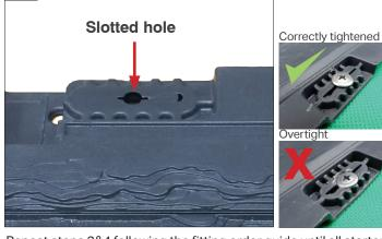
Repeat steps 3&4 following the fitting order guide until all starter strips are in place and are correctly fitted. Once correct, fully fix through slotted holes along the starter strips for permanent fix.
