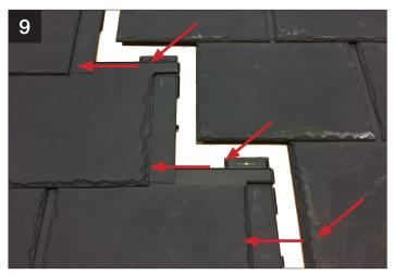
To slot the tiles together a down and left action is used in one movement. Make sure all tabs have interlocked. Tiles are fitted to the roof from left to right bottom to top. Repeat steps 7, 8 and 9 for entire layer.
