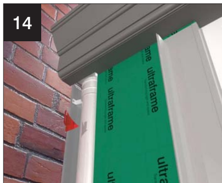
14 Fit concealed rainwater downpipe (if ordered)
