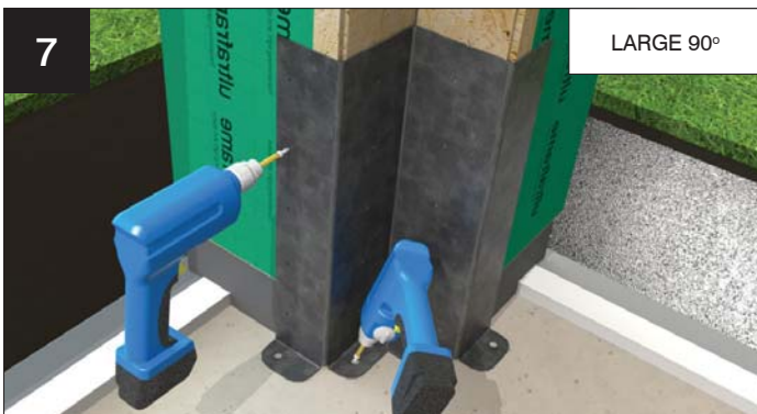
If using full height columns on a cill, remove set out post and fix internal support bracket. Large 90° column shown. Fix to column using 20 No. 5.0 x 50mm ss screws and down to floor using 4No M8 x 80mm bolts supplied. NOTE: IF FIXING TO FINISHED FLOOR LEVEL, SUPPORT SHOE MAY NEED TO BE SET INTO FLOOR.
