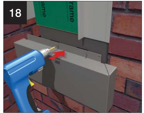
18 Screw cut down column plinth to column using screws provided. If column plinth is against frames, fit endcaps as shown in previous images. NOTE: SILICONE SEAL TOP OF PLINTH (OVER PACKERS) TO BASE OF COLUMN
