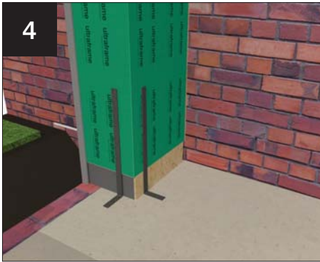
Abutment column fixing straps.
